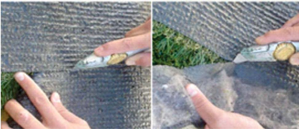
Ensure the grain in the fibres of all the pieces of turf are running in the same direction. Lift and position the turf on the prepared subsoil (do not drag into place) keeping the roll edges as close together as possible.
