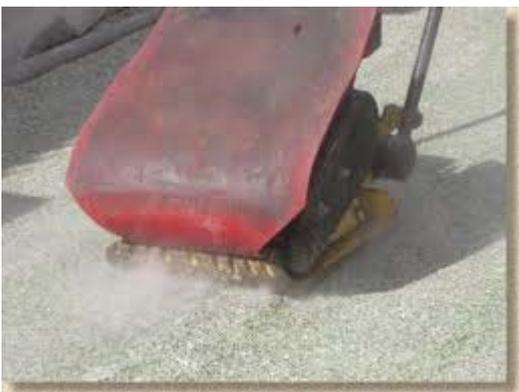
Ideally, the subsoil will be pitched slightly towards the best direction to allow for water drainage to run-off. It is recommended that edging (eg: timber, brick or stone) be installed on the perimeter of the area you want to cover with Artificial Turf, which will further secure the solidity of the area. The top level of the edging should be at the desired finished elevation, so as to avoid pooling of water.
